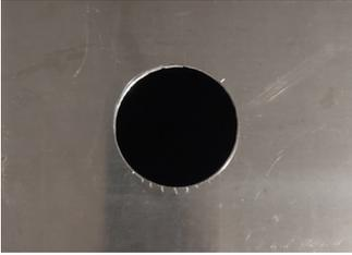
1. Locate existing hole from existing DP gauge installation in metal panel. If no hole, cut a 2-1/4" clearance hole.
