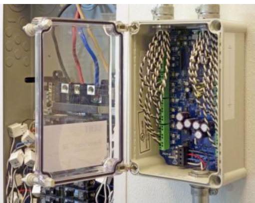
Power Squad mounted in a NEMA-rated box near electrical panel
